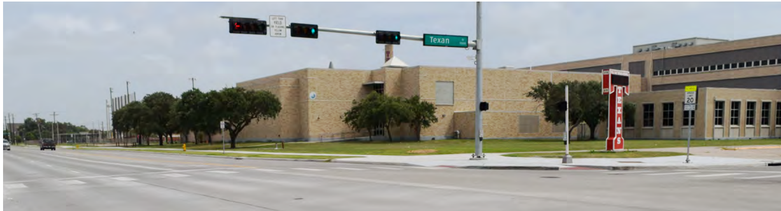
Staples St. improved under the Bond 2018 program.
